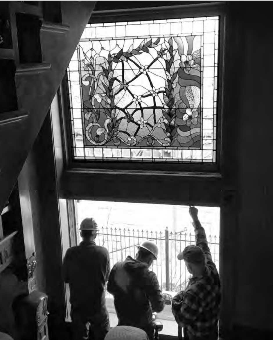
Stained glass being reinstalled at the Molly Brown House Museum by the Watkins Stained Glass Studio
