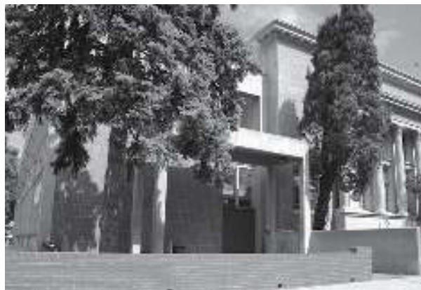
Roof Restoration at Althea Center (1955 addition in the foreground).
