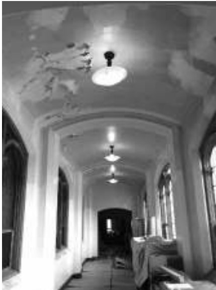
Montview Boulevard Presbyterian Church Miller Center hallway with visible peeling plaster. Photo: Shannon Schaefer Stage
