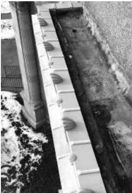
Terra Cotta restoration on the upper capped parapet. Photo: Hoehn Architects
