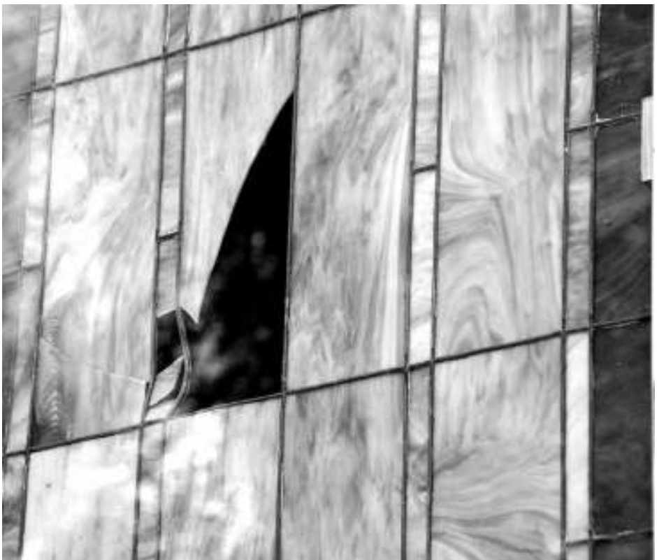
Capitol Heights Presbyterian Church, west façade stained glass damage and deterioration. Photo: Shannon Schaefer Stage, 2021
