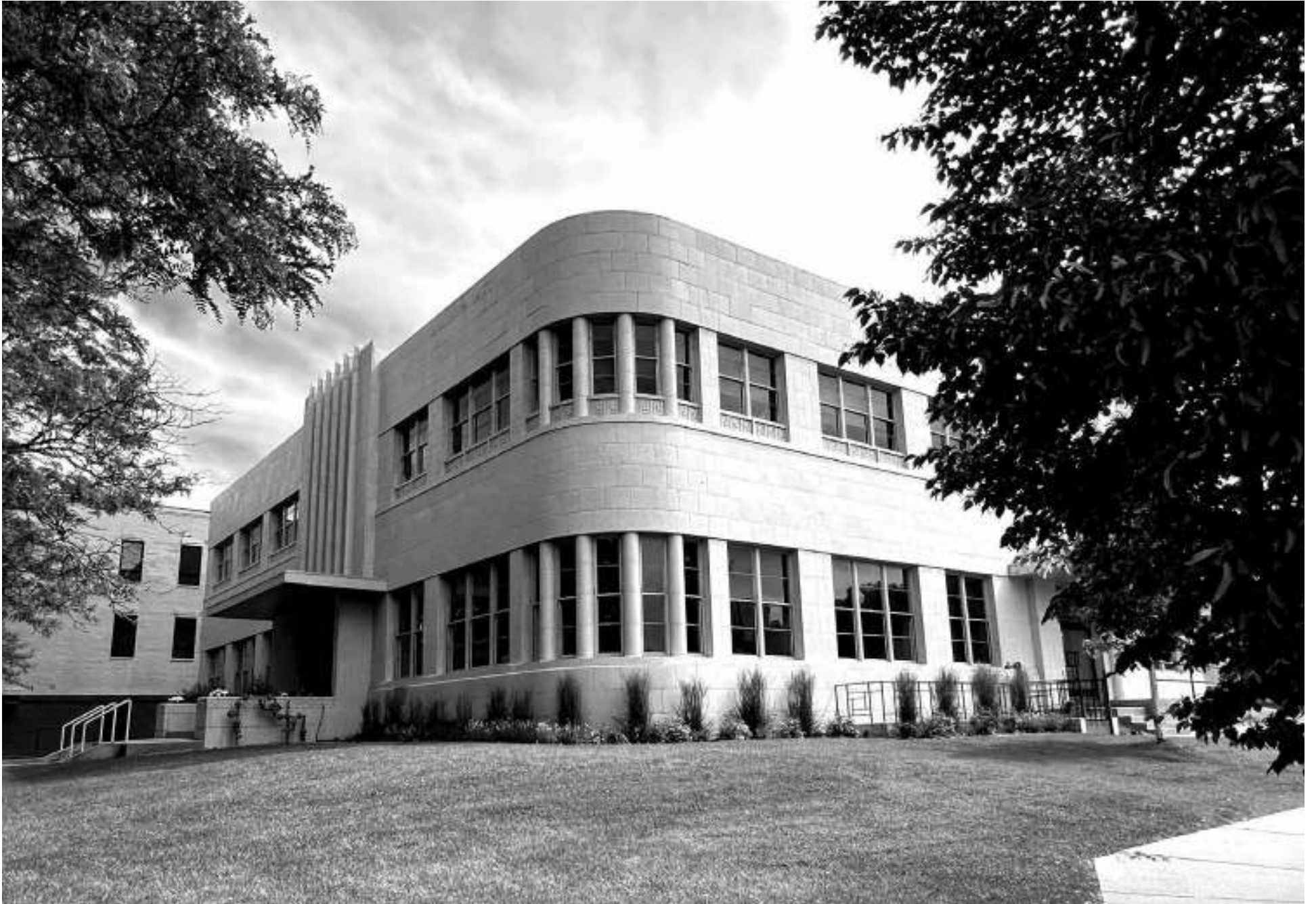
The American Woodmen's Life Building at 21st and Downing streets was designed by Denver architect Gordon White. It was built in 1950 and became a Denver Landmark in 2009. The American Woodmen was a fraternal society that provided home mortgages and life insurance to African Americans.
