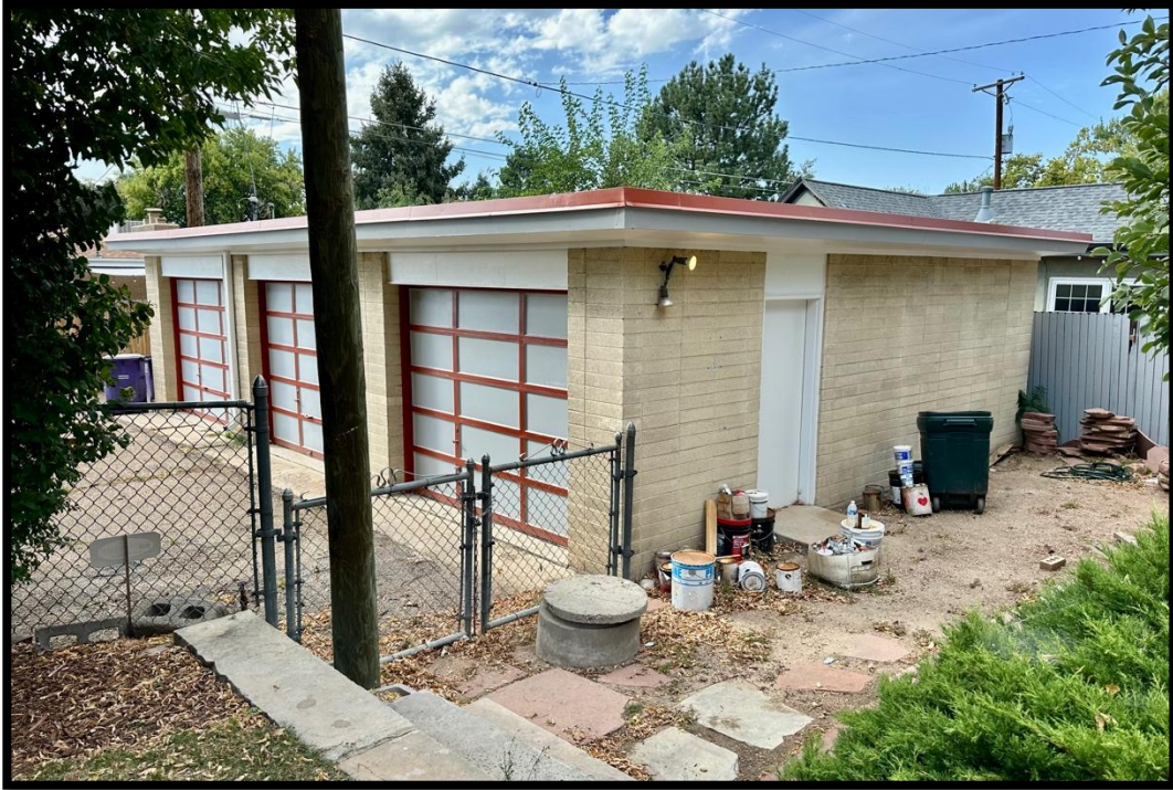
Detached Garage, View to the Northwest
