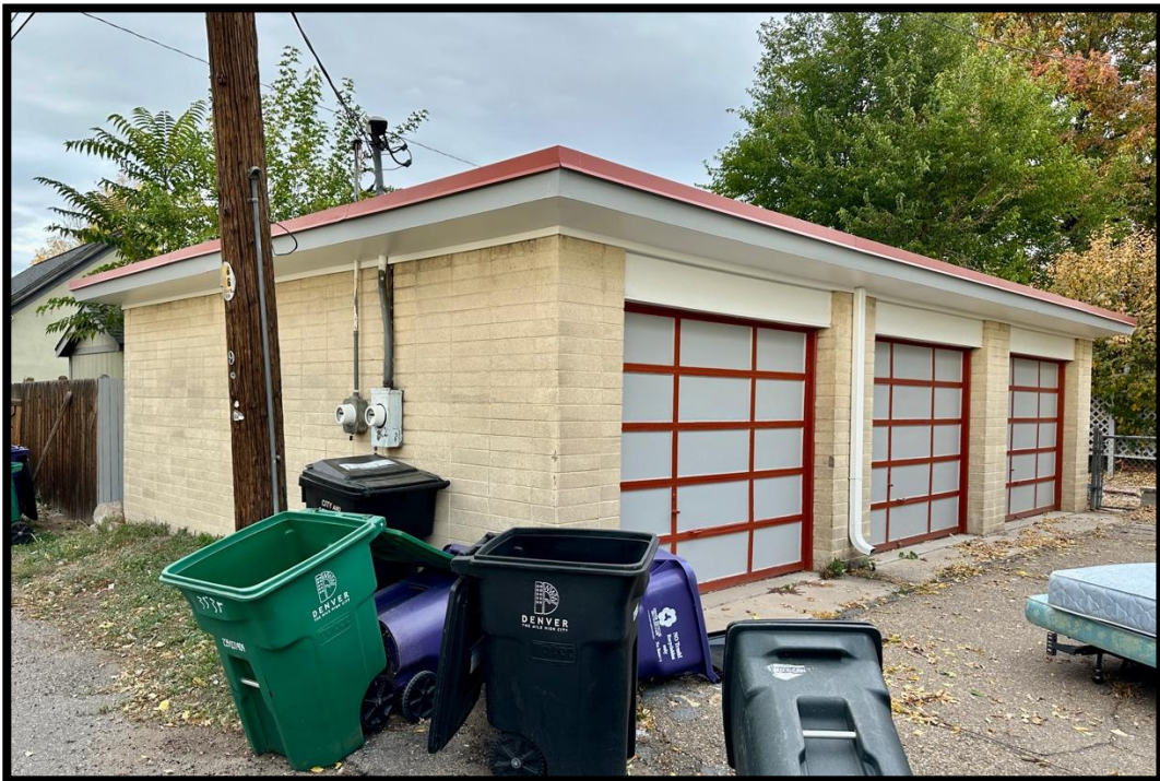
Detached Garage, View to the Northeast
