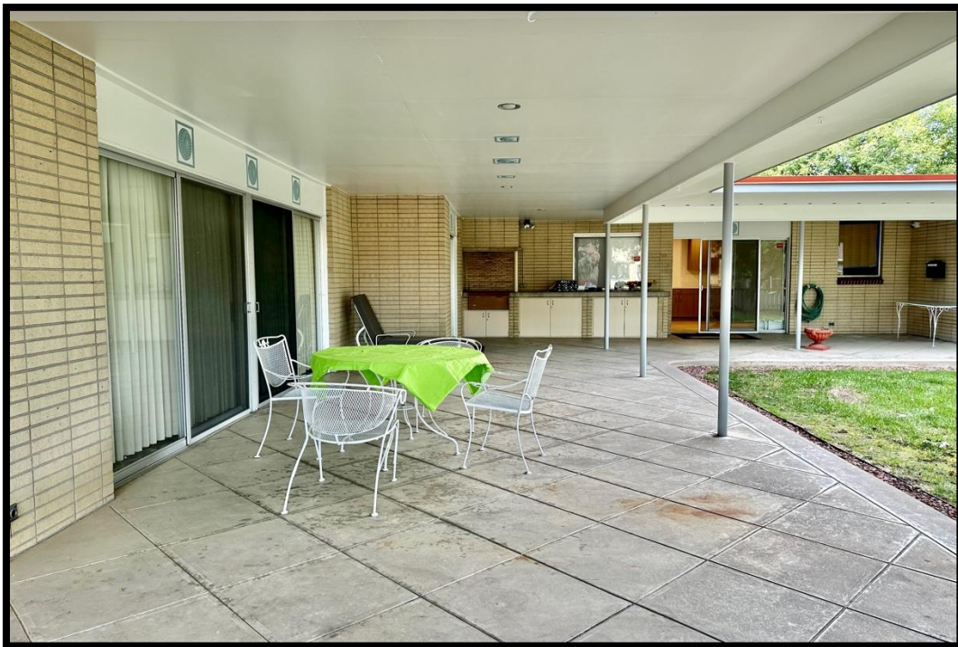
The Northeast Porch, View to the West
