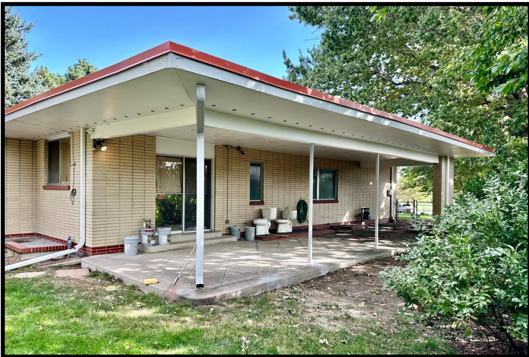
The West Porch, View to the Southeast
