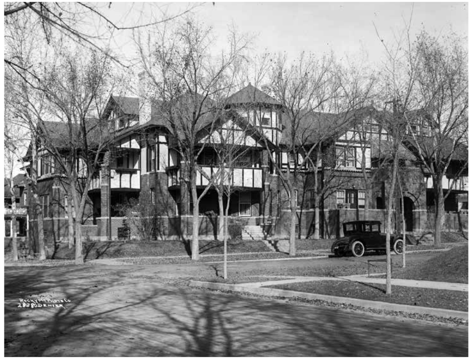
The Gables at 11th and Lafayette were originally two single-family homes that were reconfigured and added onto in the 1910s to create 14 residential units. Photo: Denver Public Library Special Collections, X- 25266
