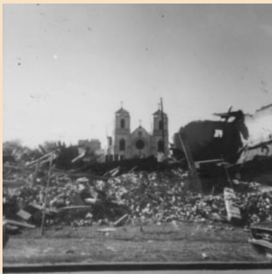
St. Cajetan's Catholic Church amid demolition, Auraria, 1973, Denver Public Library
